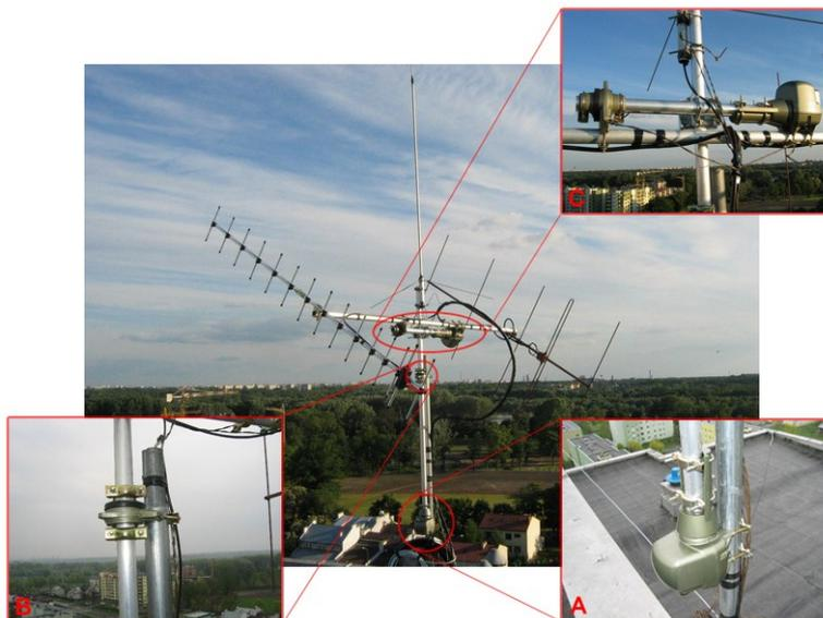
Figure 7. RC\_FNQ rotor (A – azimuth rotator, B – azimuth support bearing, C – elevation rotator with support bearing)
